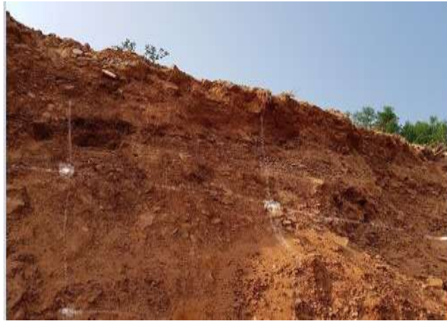
Figure 1: Marking of drill locations on the slope
